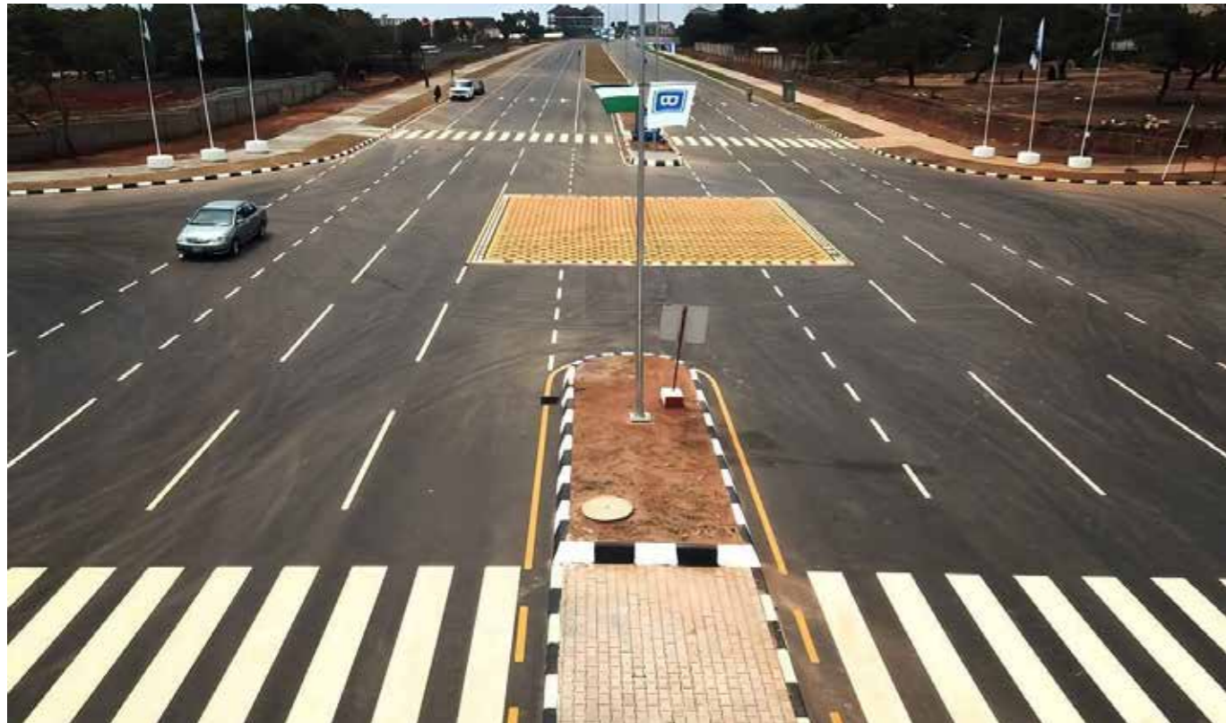
President Bola Ahmed Tinubu, ably represented by the Secretary to the Government of the Federation, Senator George Akume, commissioned the newly constructed 8-lane Arterial Road N5 (Obafemi Awolowo Way) from Life Camp Junction to Ring Road 3 (RR3).
